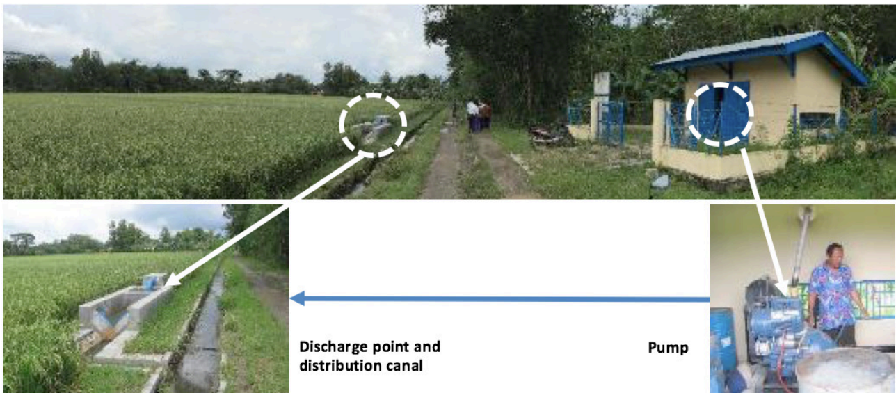
Figure 52. Groundwater bore wells for supplementary irrigation in rice field in Indonesia (GP-5.4i)
