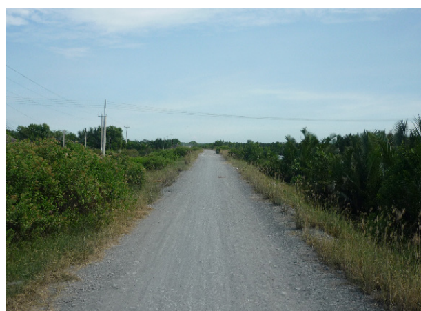
Figure 37. Polder dike including height for sea water level rise for protecting delta area of the Mekong River in Ben Tre Province, Viet Nam (GP-5.3c) Source: JICA Project Team
