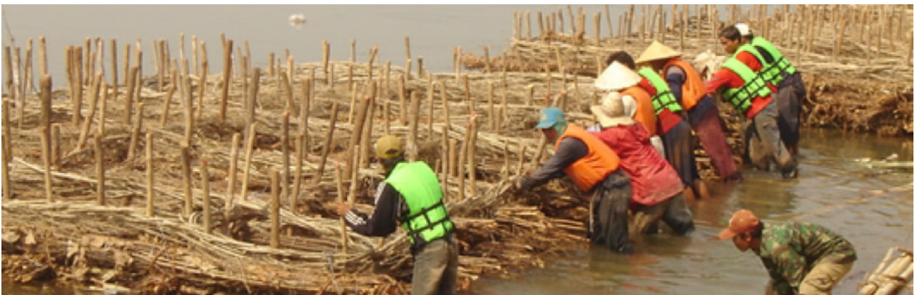
Figure 41. Riverbank protection using the Soda method, Lao PDR (GP-5.3g)
